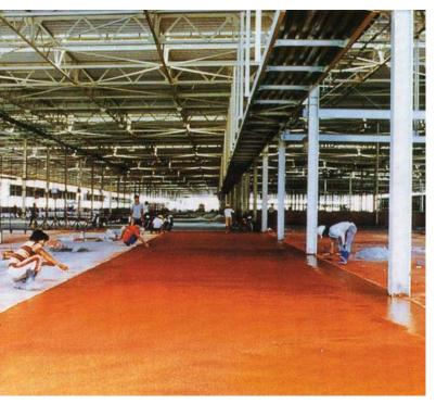
Masterpav Non - Metallic Floor Hardener is a ready to use, dry shake silica quartz mineral aggregate suitable for both interior and exterior concrete floors where areas require additional wear resistance such as:
